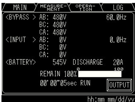
Figure 4-7 Battery Operation Values
