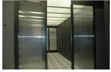
**Site #4**Cold Aisle Containment with PolarPlex Drop-Away Panels and Auto-closing Sliding Doors.
