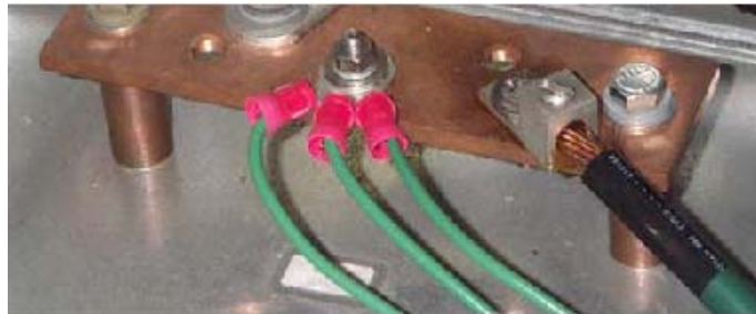
Figure 54 – S5 Grounding Example
